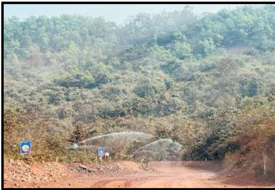
Fixed water sprinkling arrangements
